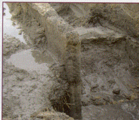
(Top) Trenchmix tool in operation (Above) Trenchmix wall excavated for inspection
