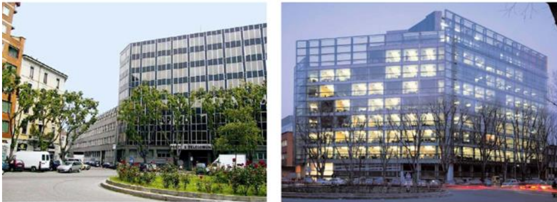
Figure 7, 8. Hines Office building in Milan before (left) and after (right) over cladding.
