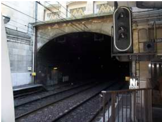
Figure 2: The metro tunnel at the station Cité Universitaire.
