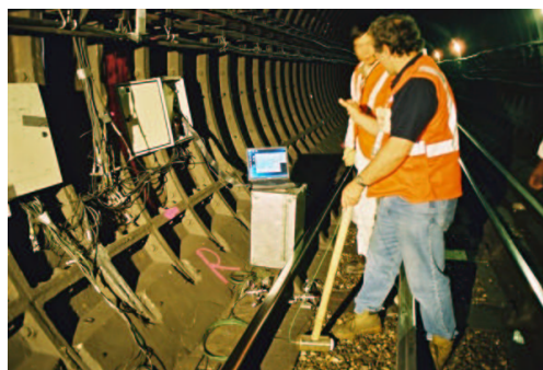
a. The Bakerloo line tunnel.
